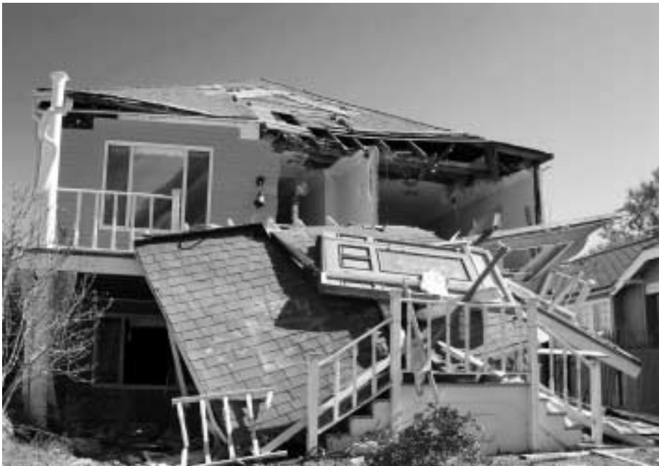
The Lakeview neighborhood of New Orleans 2 months after Hurricane Katrina. This house is on West End Blvd., just blocks from the 300 ft. levee breach on the 17th Street Canal. The area was flooded with over 12 ft. of water and sat submerged for weeks. They are not projected to have electricity until March or later.
